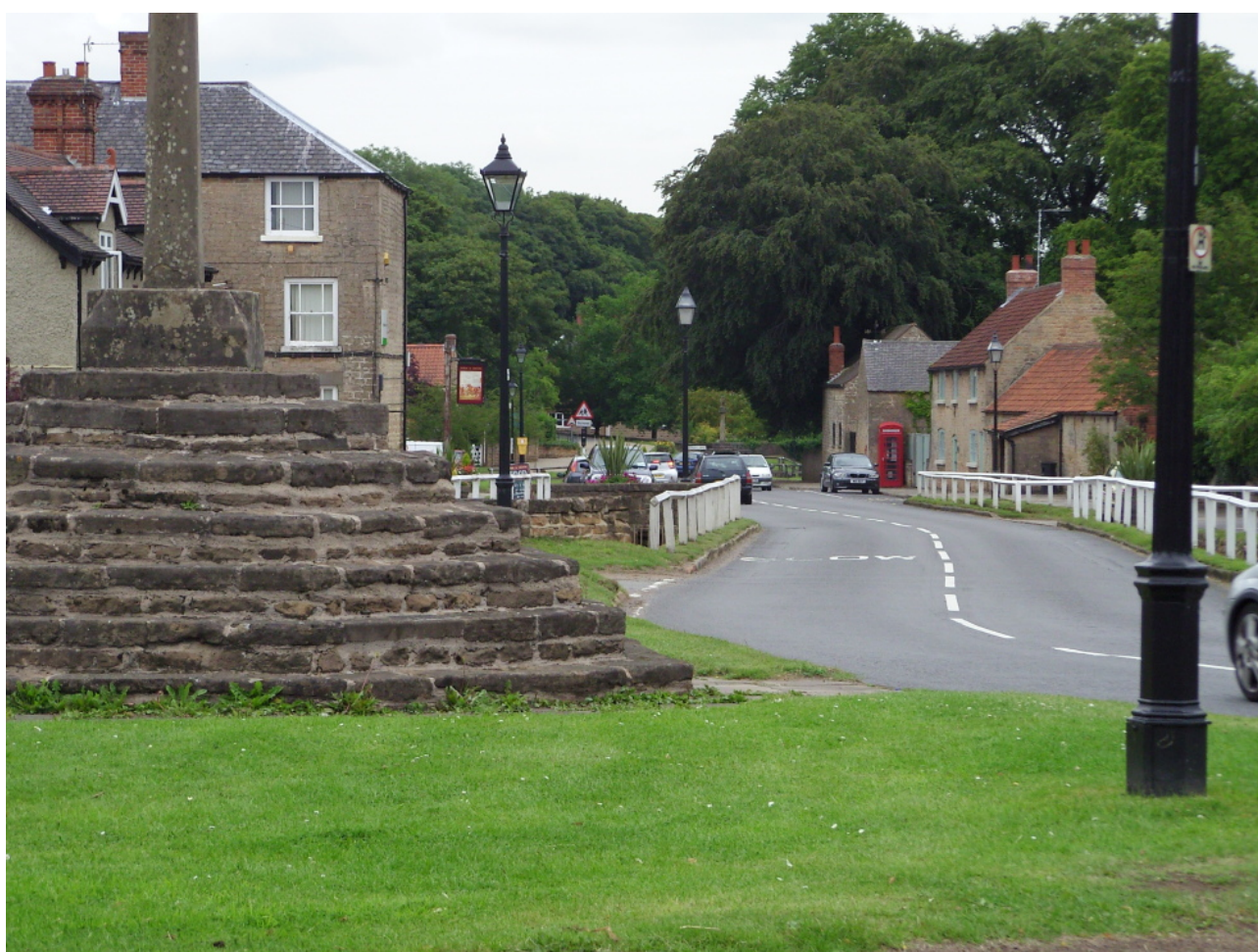
Looking east from Top Cross, the view is closed by Bottom Cross, mature trees and boundary walls
