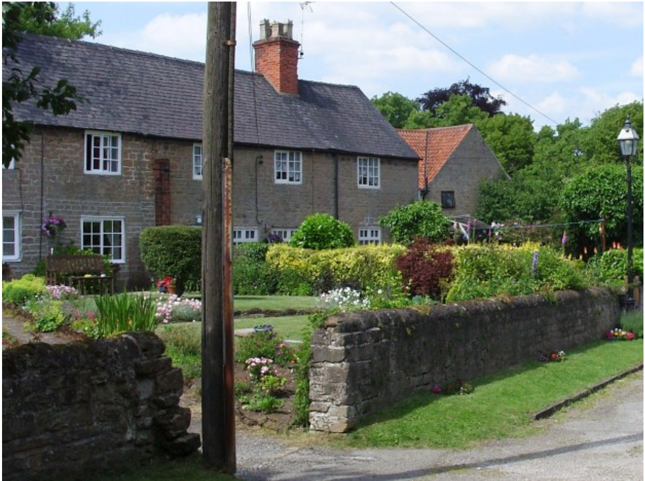
Terraced cottages with 'new' roof coverings
