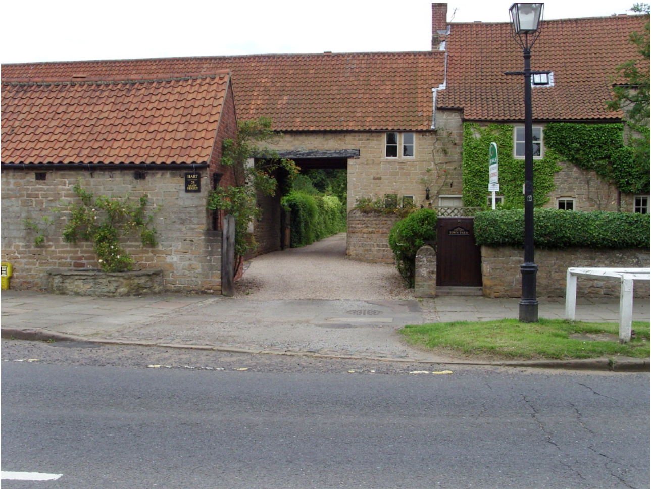
Glimpse through cart entrance at Town Farm
