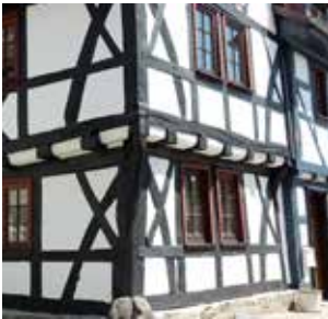
"Wild man" on the corner of this house in the street Meyersgasse
