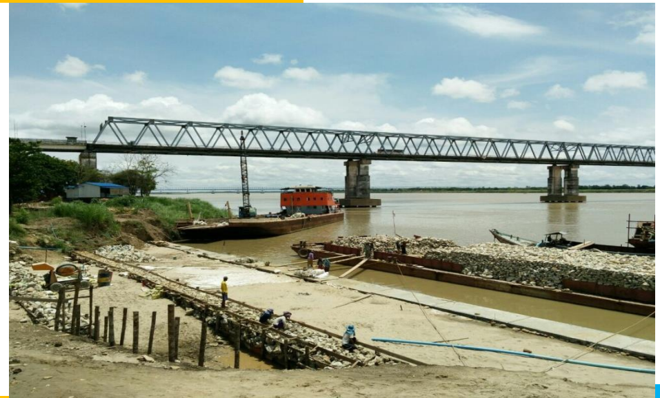
Steel basket based revetment (225 ft) under struction
