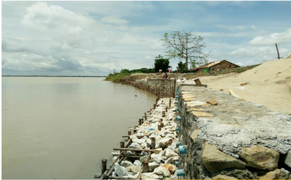
Bored pile R.W (615 ft) under construction
