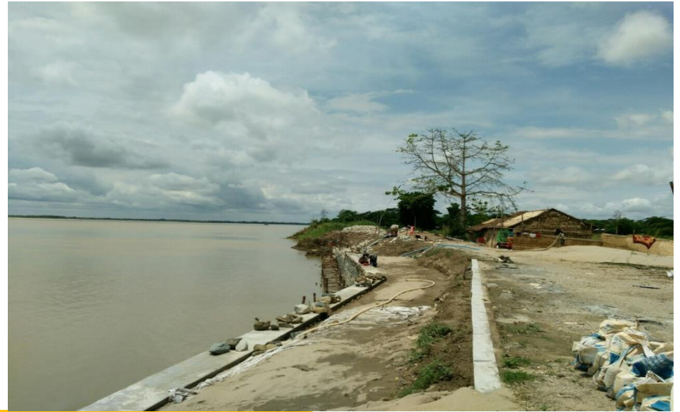
Bored pile R.W (615 ft) under construction
