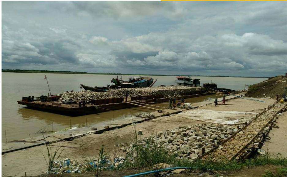
Steel basket based revetment (225 ft) under struction
