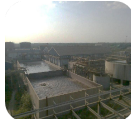
Effluent treatment Plant
