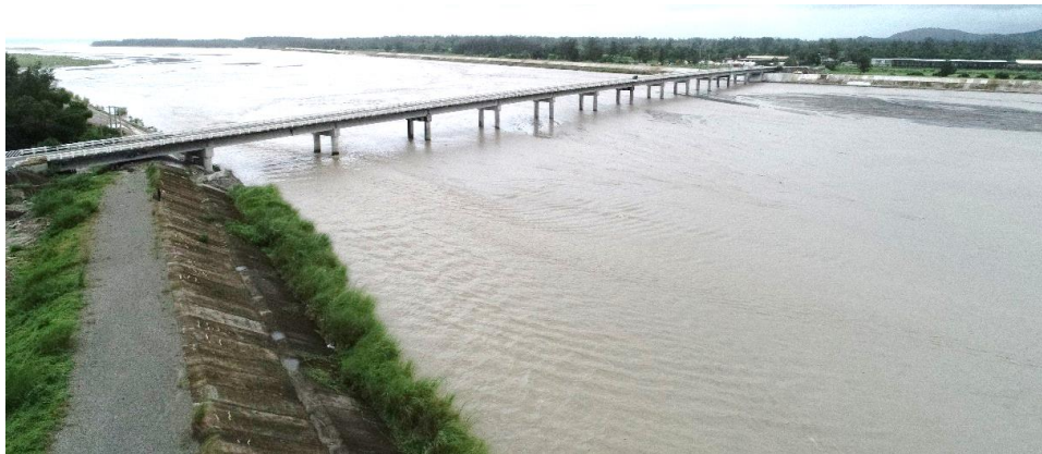
Figure 4. Existing condition of the Santo Tomas River (photo taken on August 9, 2019)
