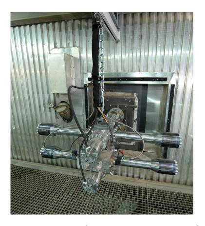
The Shock Pulse Generator TwinL is mounted at the 2<sup>nd</sup> pass and cleans the 2<sup>nd</sup> and 3<sup>rd</sup> pass.
