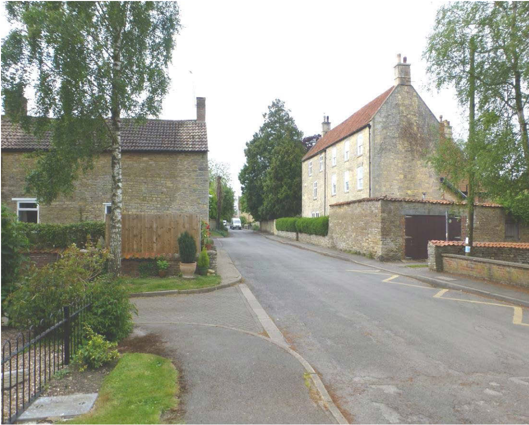
High Street looking south
