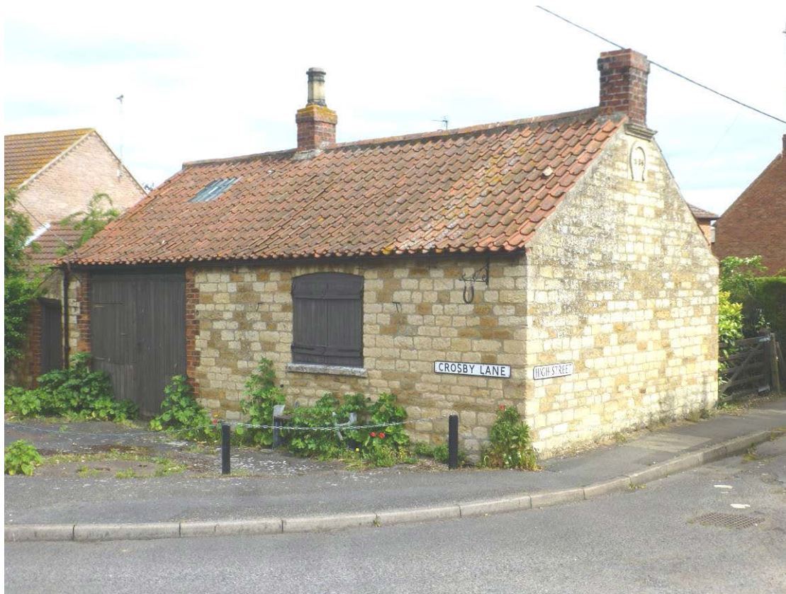
The former Blacksmith's Forge and Farrier's Workshop
