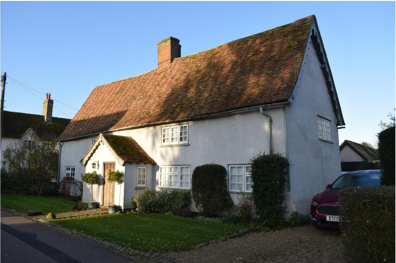
Figure 2.1: The White House (1102690) on Chapel Street.
