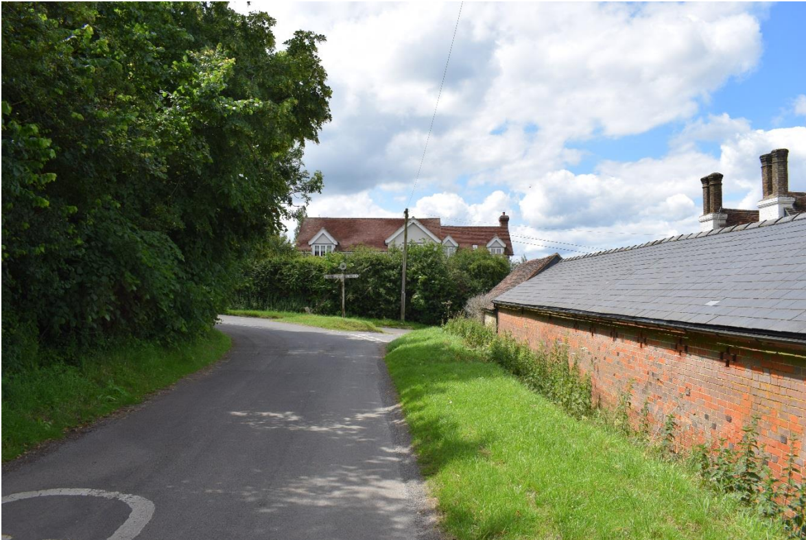
Figure 2.1 View of the low, red brick barn associated with Partridge Hall Farm fronting an unnamed lane entering the Conservation Area from the north-east. The octagonal external stacks of Partridge Hall Farm Cottage (1176567) are in the background, on the right (looking west).
