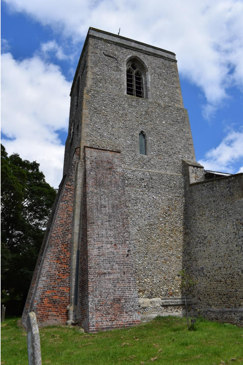
Figure 2.3 The Grade I listed 14 th century Church of All Saints (1176178), including the heavy 17 th century phase of red brick buttressing applied to its tower (looking north).
