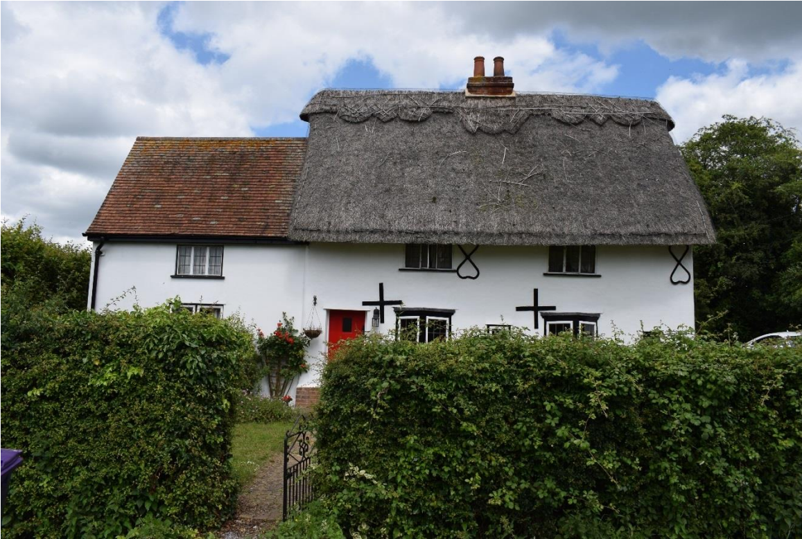
Figure 2.6 The Grade II listed late 17 th century Walnut Tree Cottage (1347363), with later extension. Along with Moss Rose Cottage, these represent two remaining examples of a cluster of post-medieval structures which once fronted Payne End (looking north).
