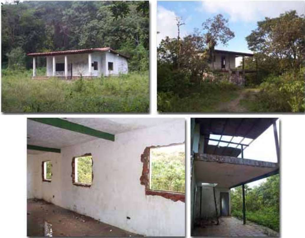
The Terepaima ranger stations are completely destroyed and are therefore not available for surveillance purposes (photos: César Aponte).
