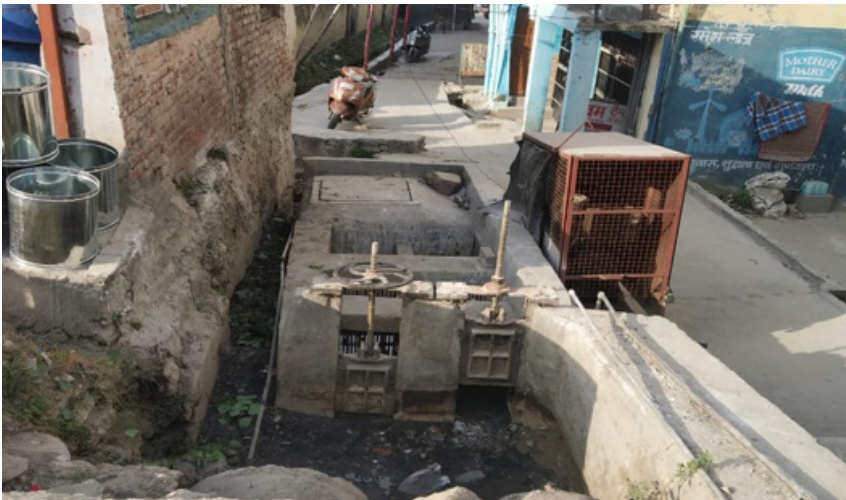
Sewage is conveyed through Nallahs after tapping
