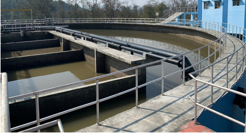
The Only STP with circular SBR tank: Motharawala STP 20 MLD, Dehradun
