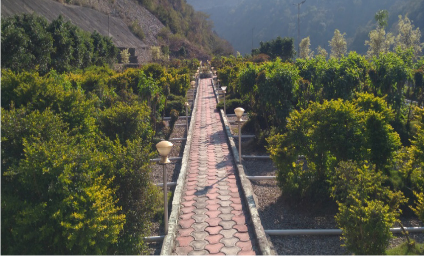
1.4 MLD Soil Based Technology STP
