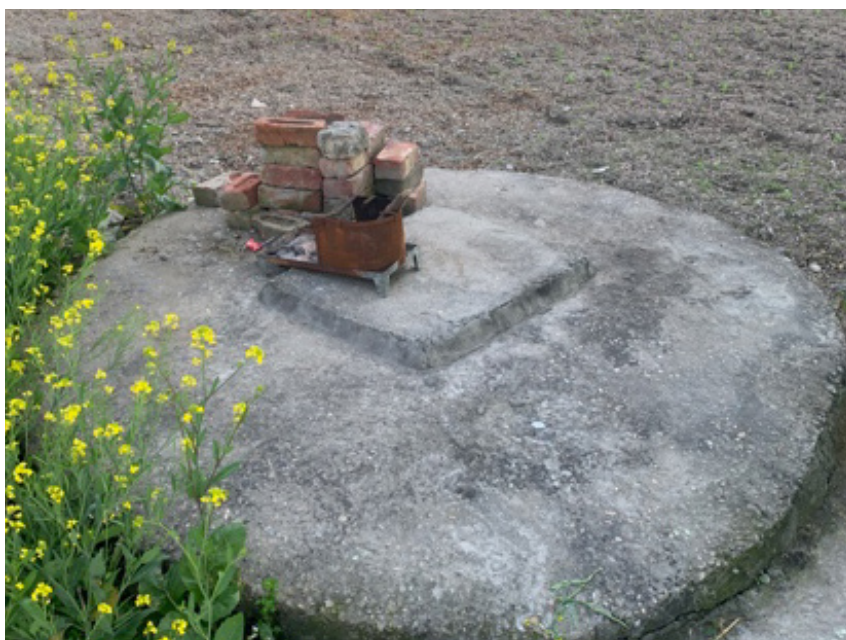
Circular pit (Onsite containment system)
