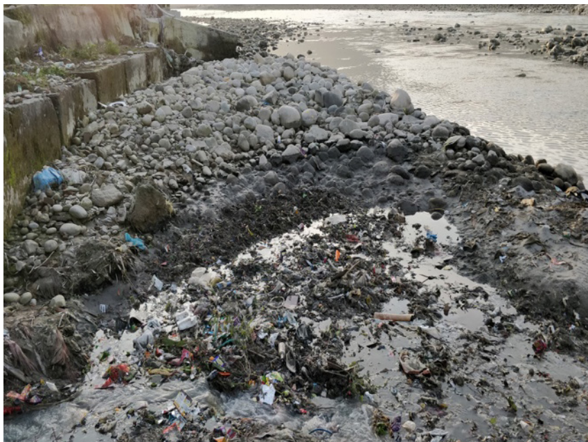
Greywater directly entering to the river through open drains
