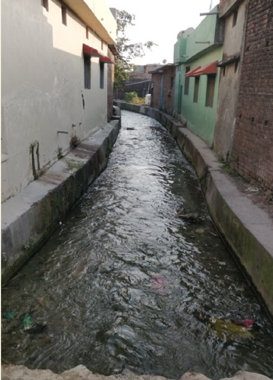
Greywater outlets from HHs into main drain
