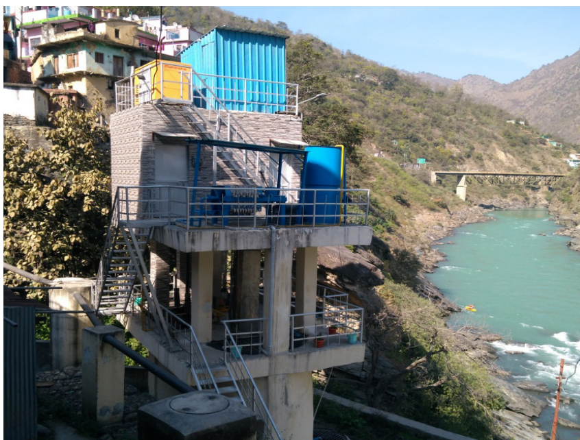
150 KLD Sequential Batch Reactor STP
