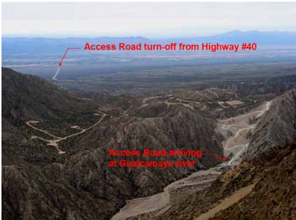
Figure 5-1 Project Primary Access Road
