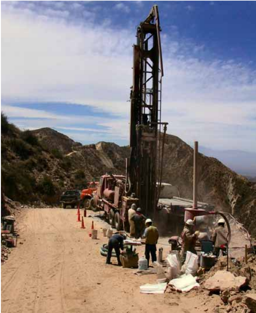
Figure 11-1 Reverse Circulation drilling at QDD
