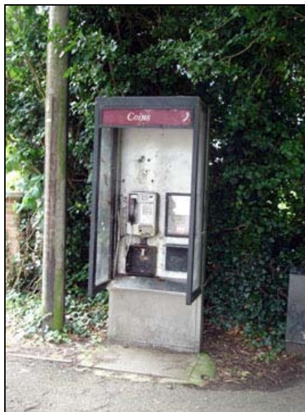
Figure 20. Vandalised redundant telephone kiosk
