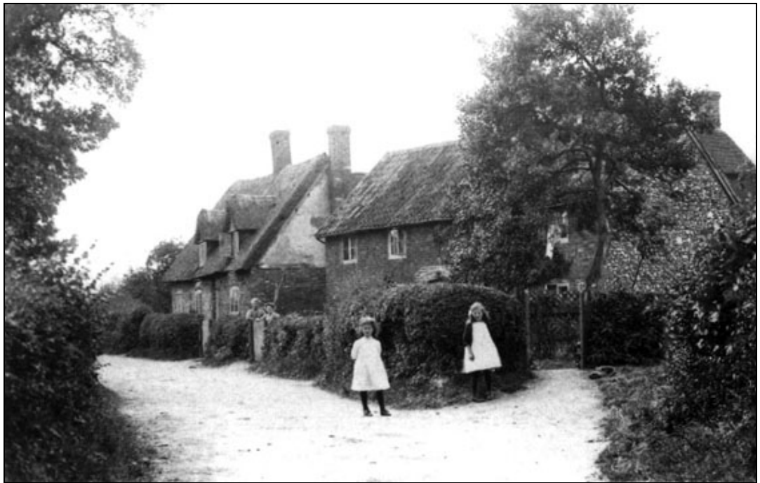
Figure 7. Fullers Mead Cottage, Mead Cottage and a brick and flint house since demolished (Ashby 2004)
