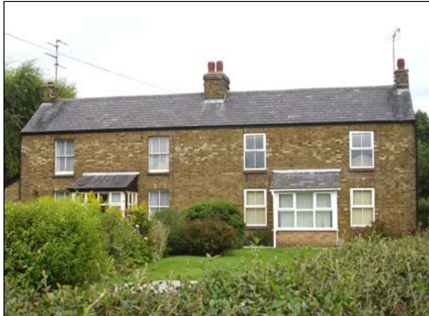
Figure 21. Pair of 19 th century cottages, one has retained its original timber sash windows, the other has uPVC replacement windows.
