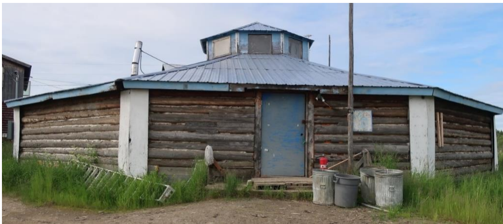
FIGURE 21 KALTAG COMMUNITY HALL
