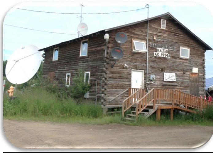
FIGURE 18 CITY OF KALTAG
