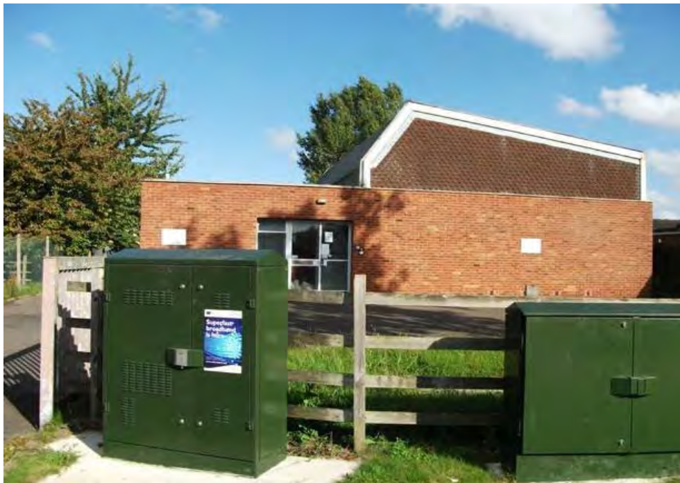
Fig 99: The telephone exchange building has an irregular-shaped roof profile finished in polygonal hanging tiles
