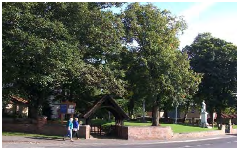
Fig 63: St Mary's Church is largely screened by vegetation in views from the village centre, but individual components of its wider setting, including the village war memorial, its lych gate and those very trees which obscure it
