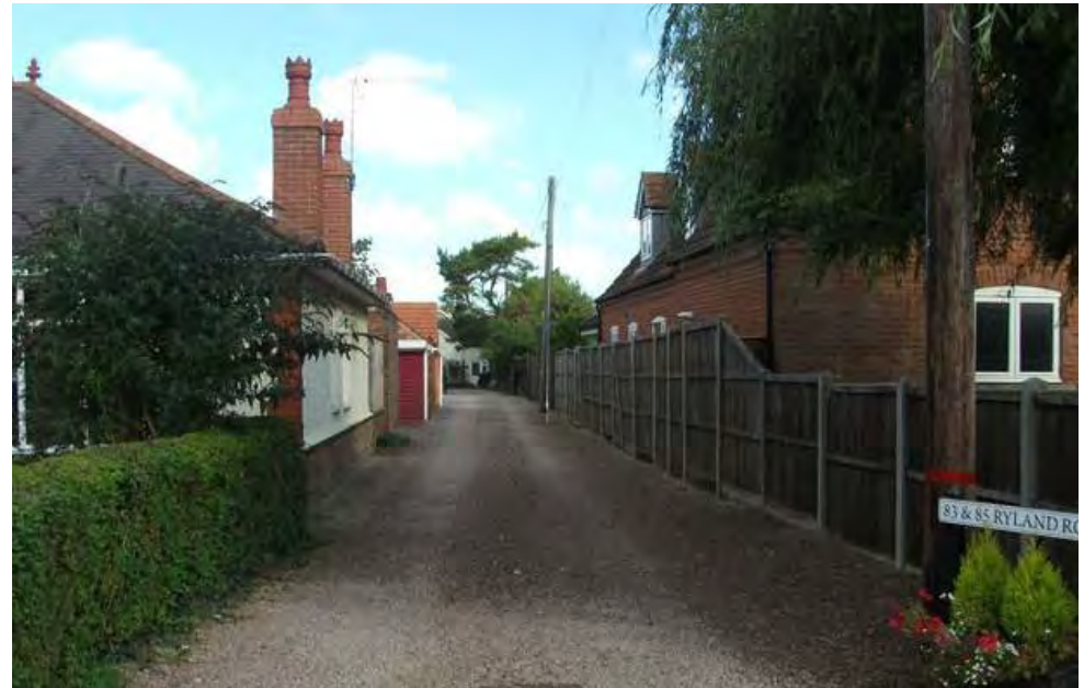
Fig 97: A number of backland developments have appeared to the north of Ryland Road
