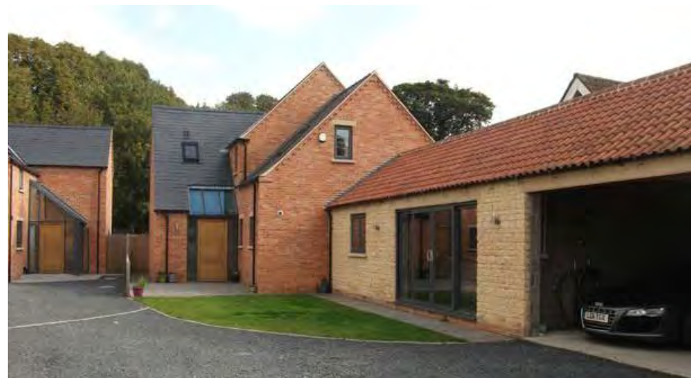
Fig 72: New development has been successfully integrated into the conservation area by drawing inspiration from local vernacular building forms and using traditional materials
