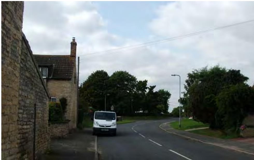
Fig 51: Looking back towards Healthlinc House, the presence of the hospital is barely perceptible due to the thick planting which encloses it
