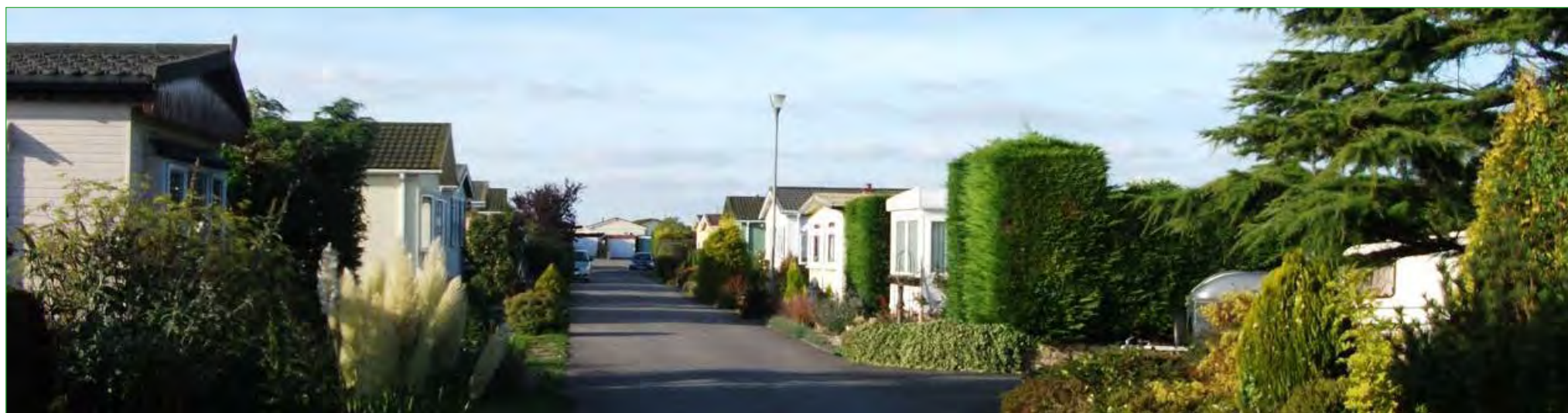
Fig 37: The linear nature of the roads and consistent spacing, positioning and orientation of the individual properties make for very well defined streets
