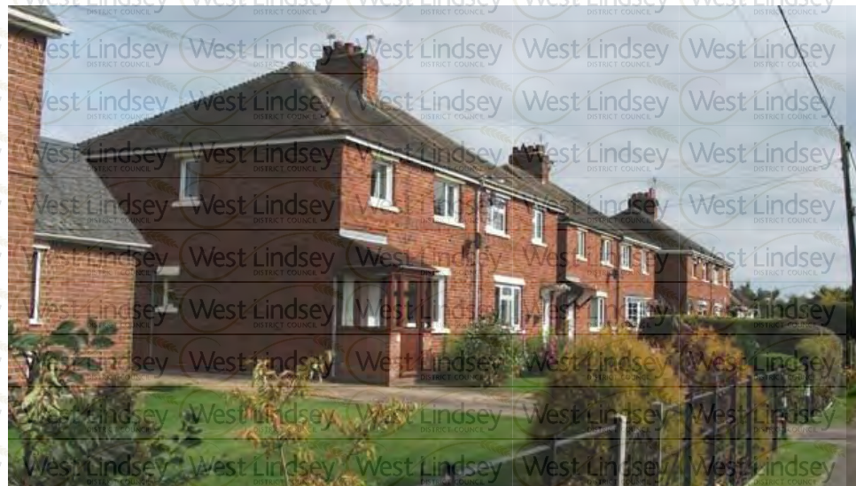
Fig 47: Red brick inter-war housing lines Cliff Road at the gateway into Welton
