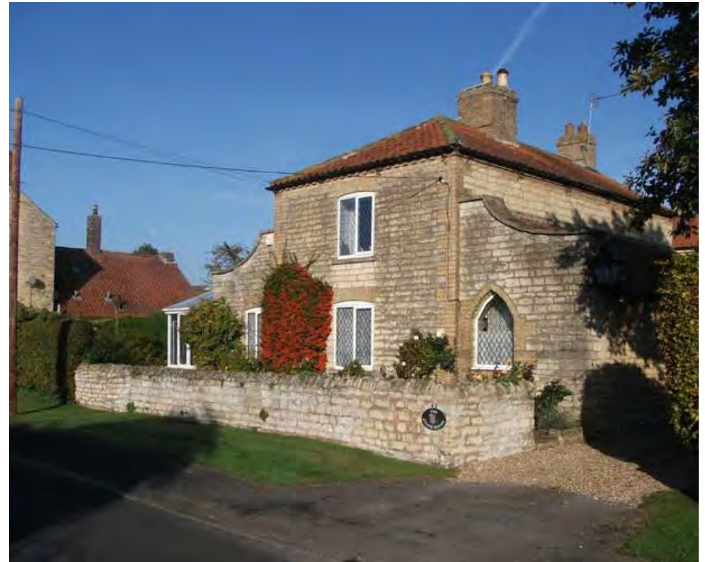
Fig 118: 63 Eastfield Lane is another characterful building where stone is the main building material, used for both the boundary walls and in the construction of the dwelling itself
