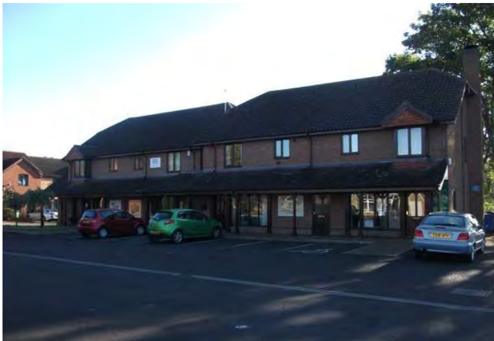
Fig 109: A parade of small shops completes the retail cluster at Ryland Bridge
