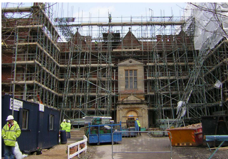
Shaw House, during restoration
