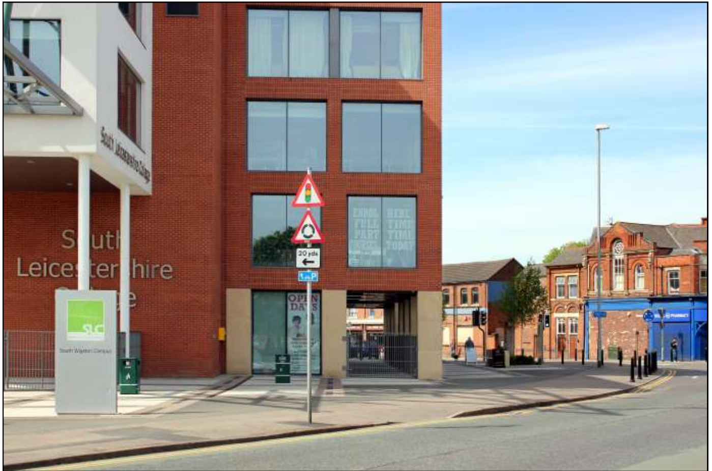
South Leicestershire College on the corner of Canal Street and Blaby Road, South Wigston. Photo Tony Danvers May 2013.
