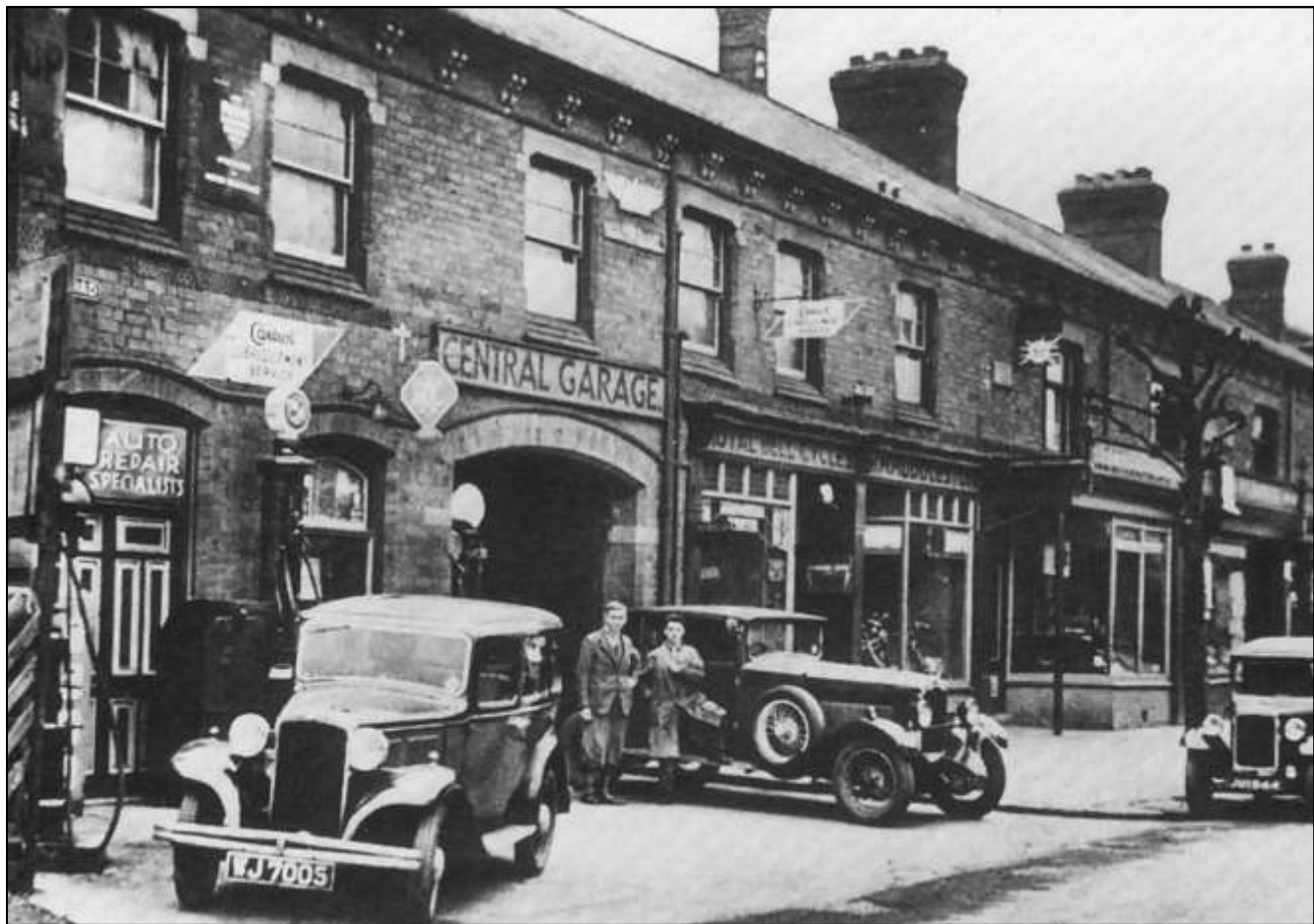
Huddleston's Garage & Bicycle Centre on Blaby Road, South Wigston, circa 1933. The garage ceased trading in the 1960's and is now the site of South Leicestershire College. See also page 70.
