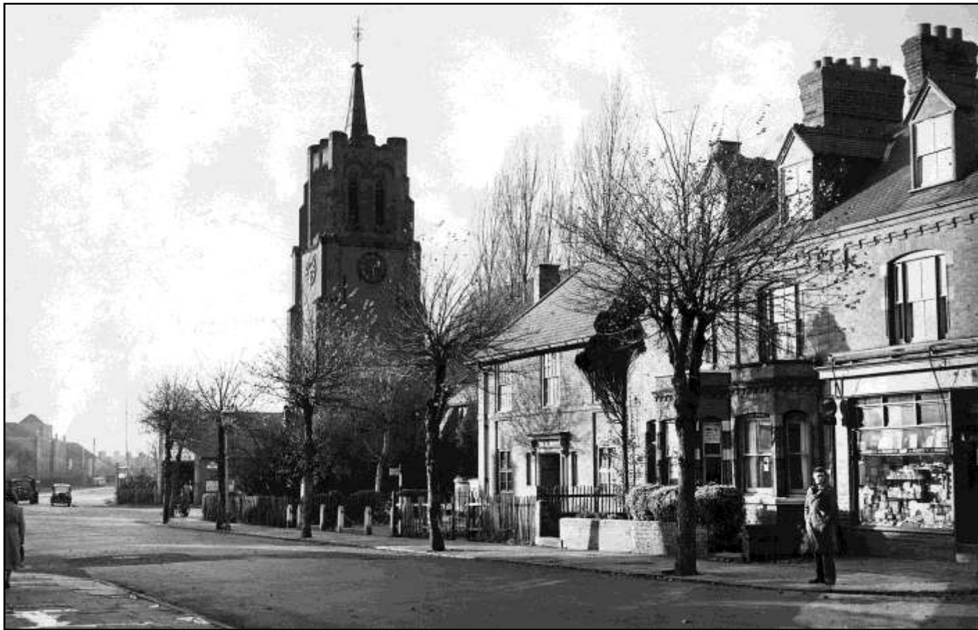
Blaby Road, South Wigston, with St. Thomas's Church in the background and the Chemist shop on the near right of the picture, circa 1940.
