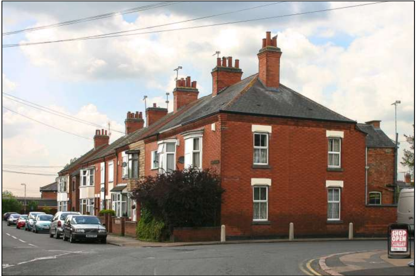
The corner of Countesthorpe Road and Railway Street, South Wigston, showing little change from the photo opposite, apart from the factory units in Park Street. Photo Kieran Smillie May 2013.
