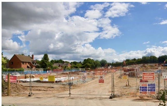
'The Racks' development being built
