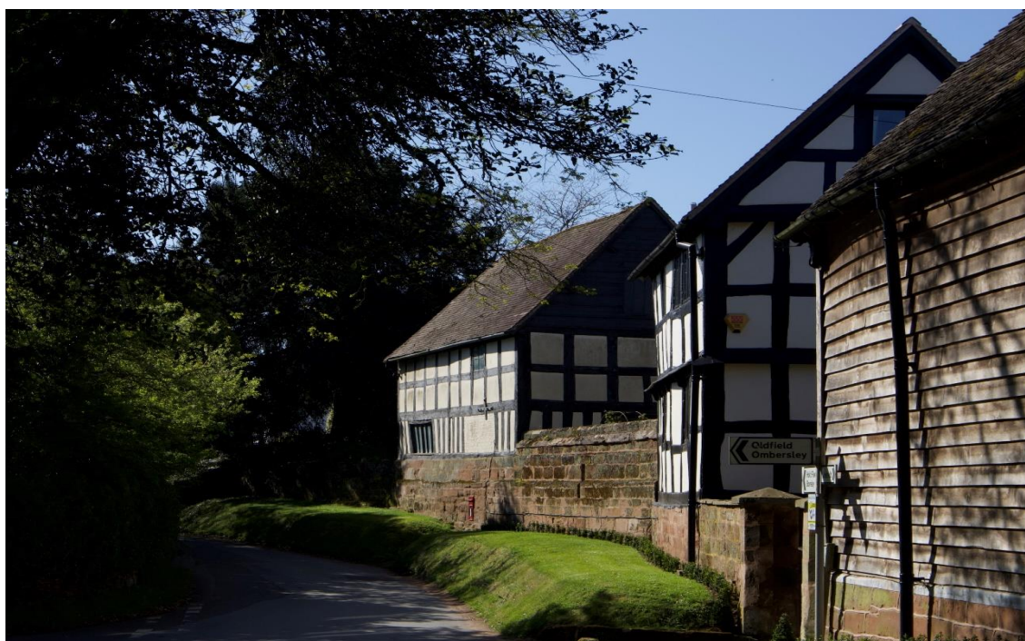
Pipestyle House and Cider Mill, Uphampton, half-timbered with typical sandstone walling
