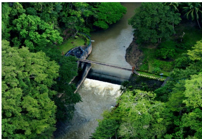
Figure 25: Tumaga River Diversion Weir
