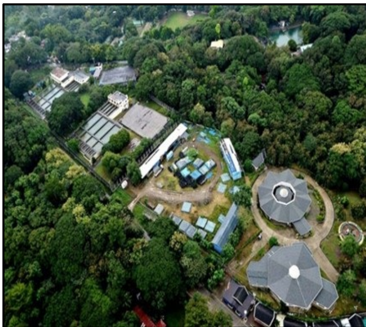
Figure 23: Aerial View of ZCWD Phases 1 and 2 Water Treatment Facilities
